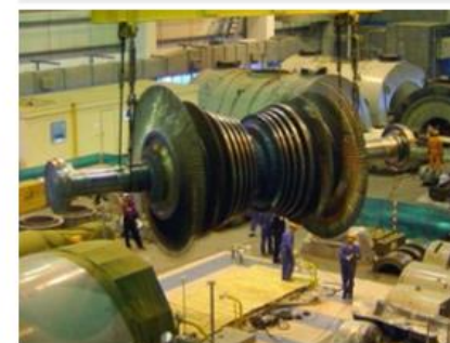
Increased maintenance costs
